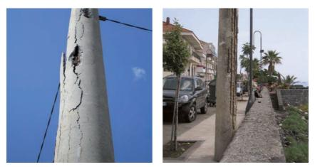
Fig. 17/18: Spalling of the concrete cover due to reinforcement corrosion (severe exposure to sea salt)
