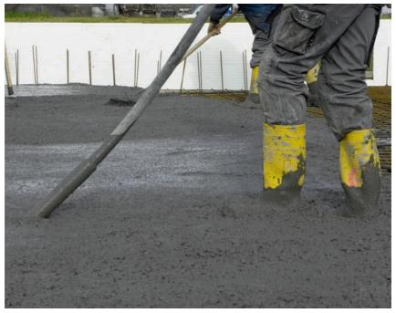
Fig. 9: Compacting the concrete with vibrating cylinder
